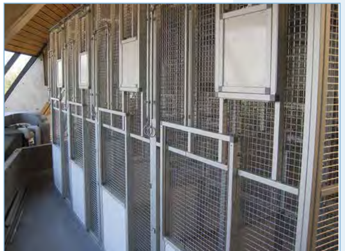
ASSINIBOINE PARK ZOO - bird holding with multiple guillotine shift doors
