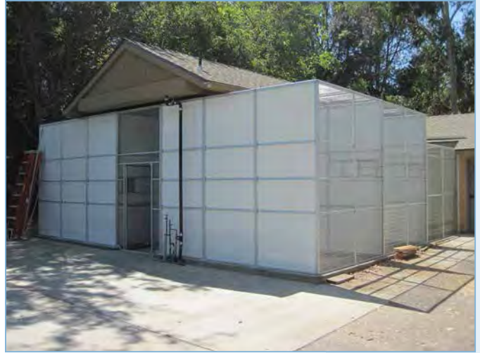
Small primate holding area
