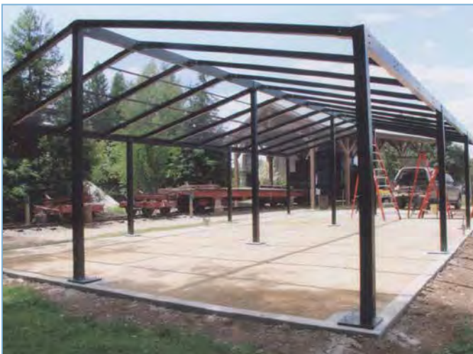
Post and beam aviary - 24'W x 45'D x 12'H, framework only
