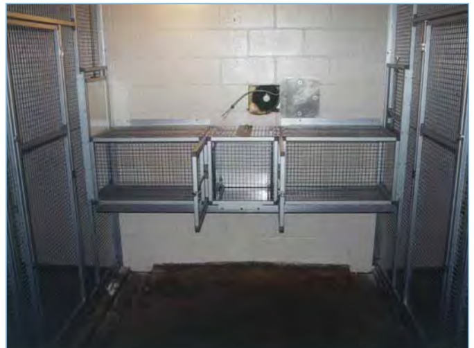
FORT WAYNE ZOO - shift tunnel with squeeze box
