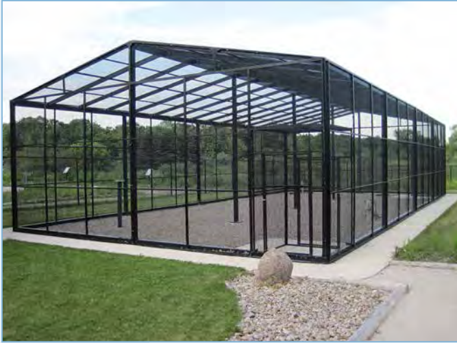
EARTH RANGERS - post and beam aviary - 30'W x 60'D x 15'H
