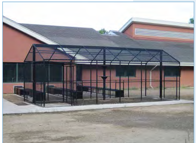
EARTH RANGERS - tunnels connecting to outdoor enclosures
