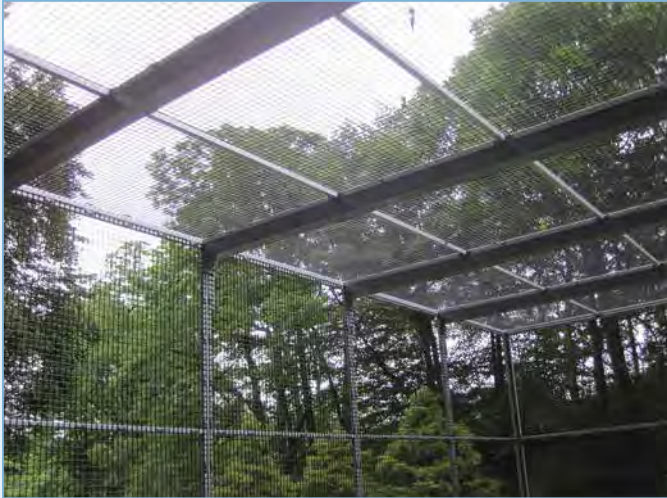
BALTIMORE ZOO - roof support beams in holding units
