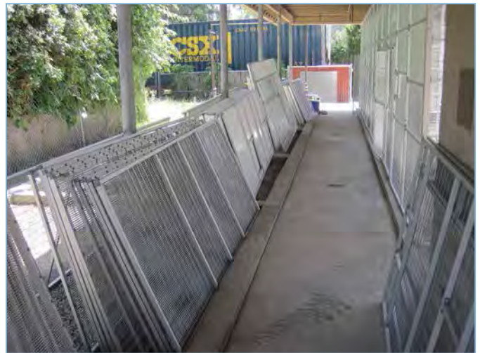
Cage panels staged for installation
