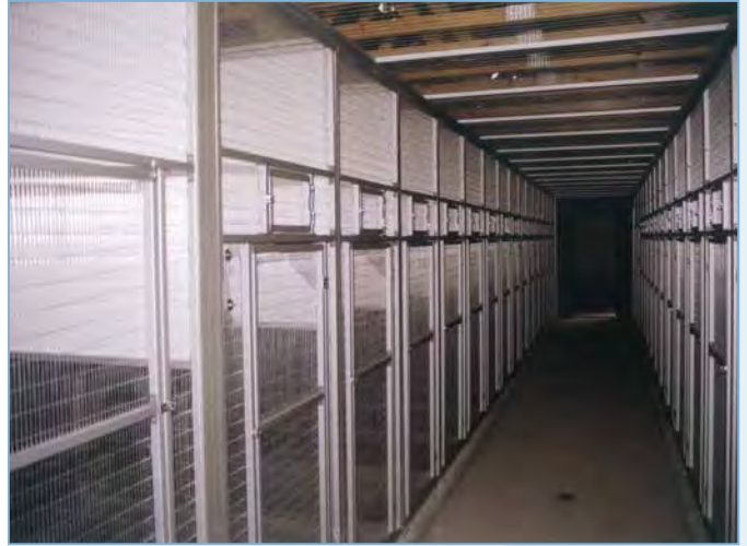
RIVERBANKS ZOO - bird holding building
