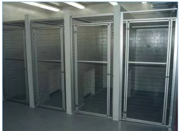
Cage fronts and tops, mounted between masonry walls
