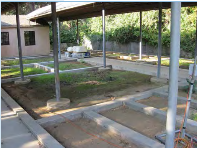
8" wide concrete curbs
