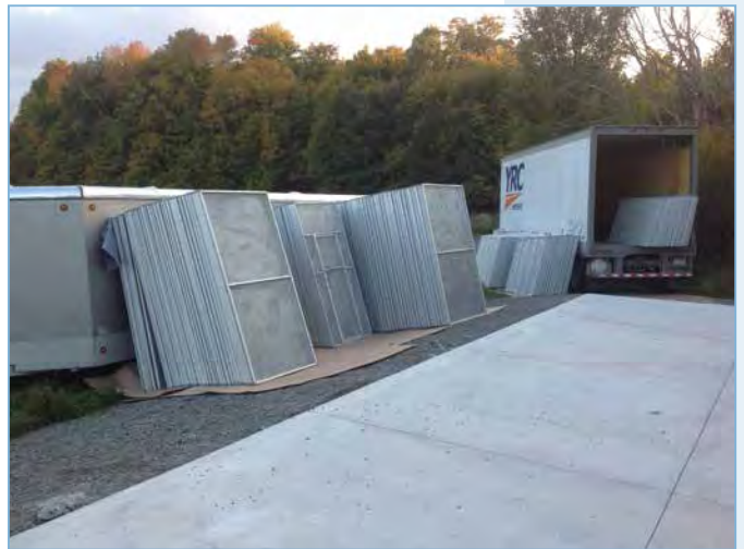
Cage panels staged, ready for installation
