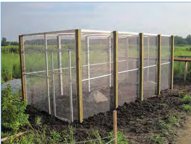
WILDLIFE DISCOVERY CENTER - flight cage with wood support posts 8'W x 20'D x 8'H
