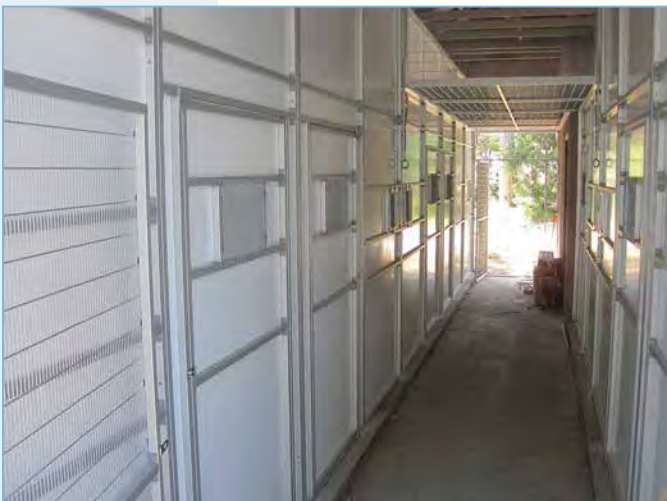
Hallway view of small primate holding
