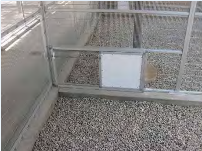
L.A. ZOO - horizontal shift door, with stainless steel pull rod
