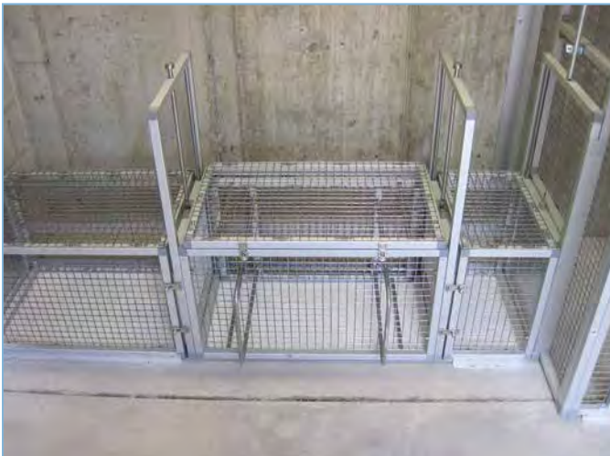
POTAWATOMI ZOO - otter tunnel and removable squeeze box
